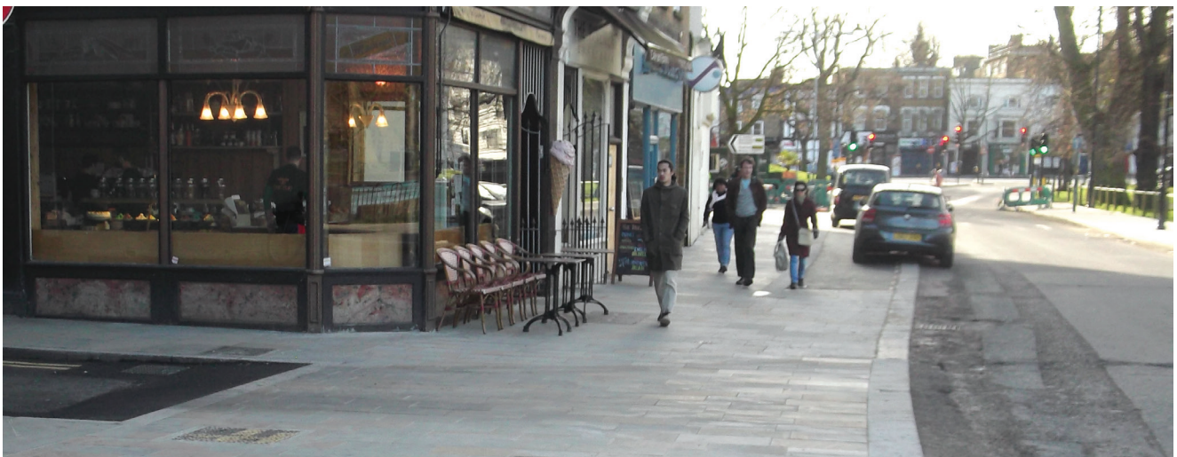
Blended junction, Bromells Road, Clapham. Footway continues across junction using slightly smaller element paving for strength
