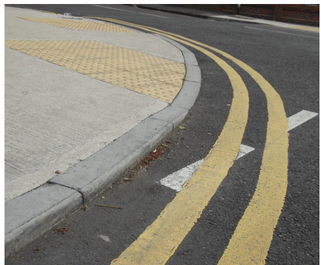
Flat-topped road hump across entire junction. Flush kerb and tactile paving provided at crossing points with upstand left elsewhere
