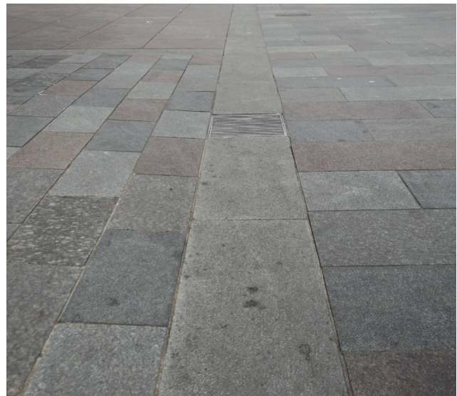
Gentle gradients and a flush channel block leading to pedestrian-friendly gully grating
