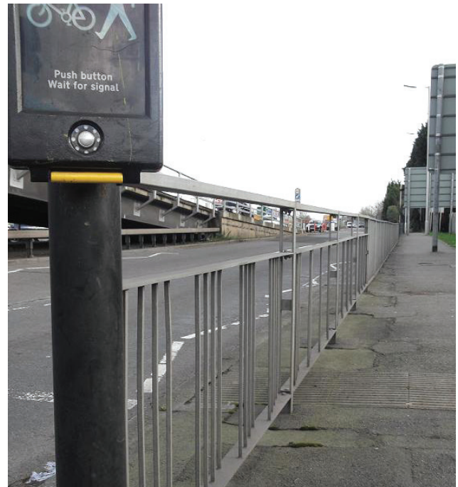
Contrast between “see-through” and non-see-through guardrail
