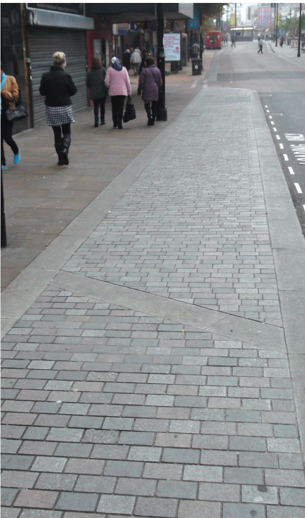
Level surface footway loading bay allows for essential servicing of shops but is fully available to pedestrians when loading is not taking place
