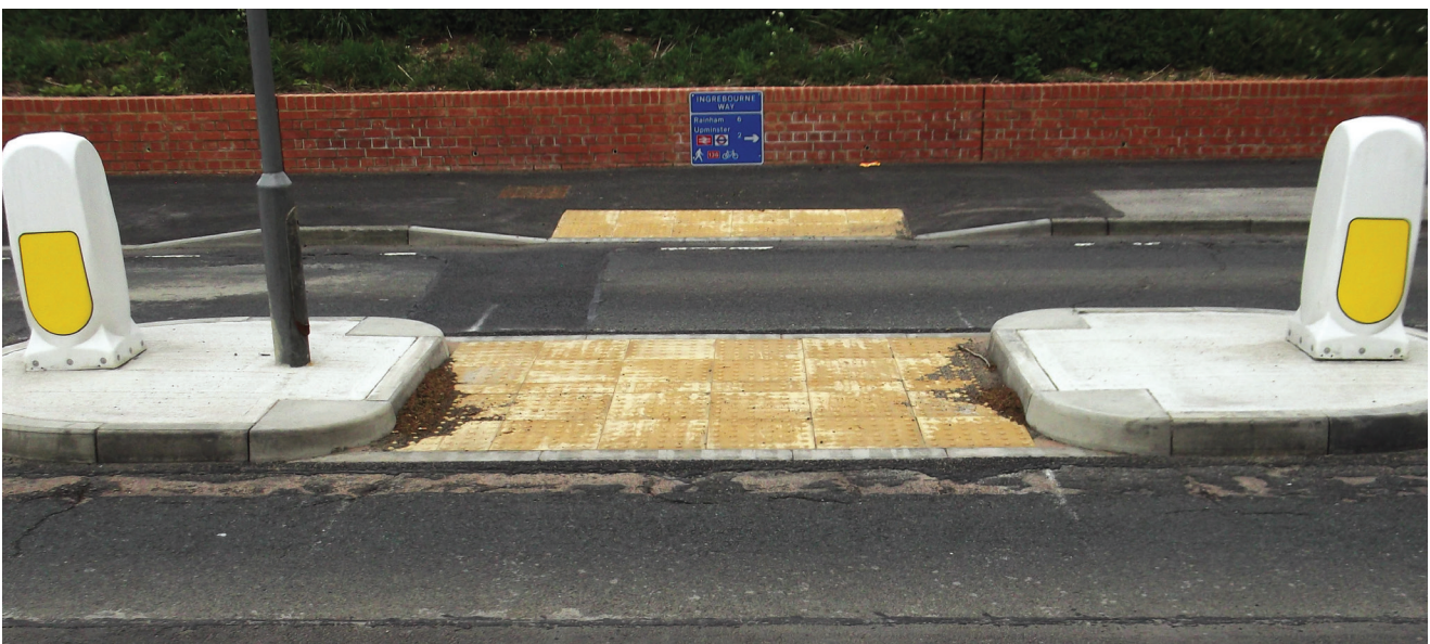
Pedestrian Refuge: wide and deep enough for use by both pedestrians and people riding bicycles
