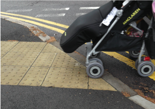
Flush dropped kerb with tactile paving and a gentle ramp
