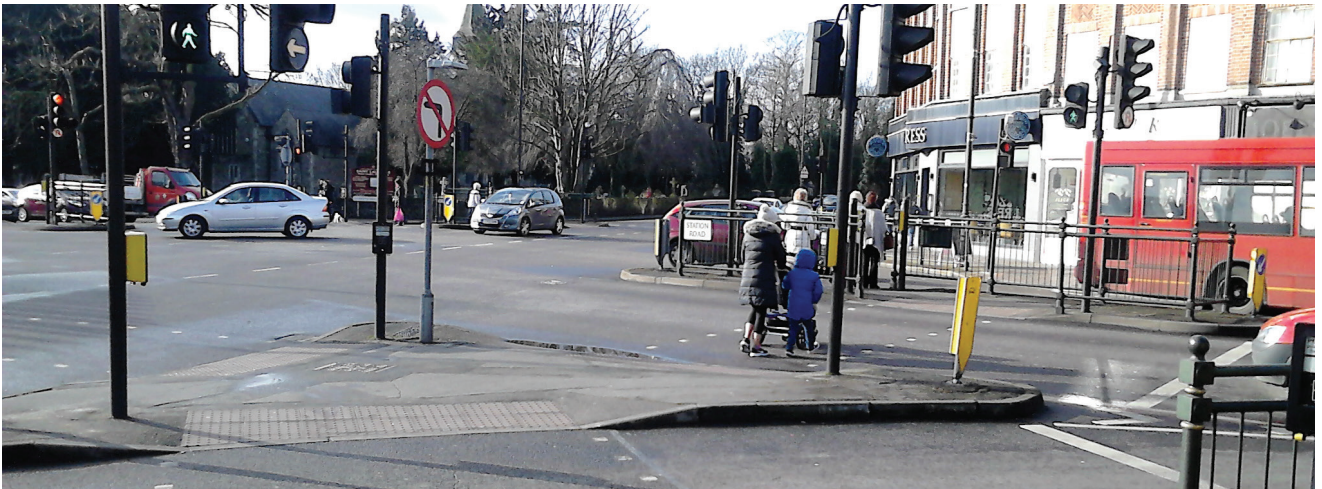
Multistage crossing at a junction
