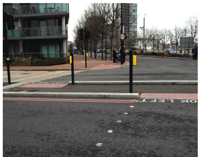
Western Gateway, Docklands: PedX crossing without guardrail
