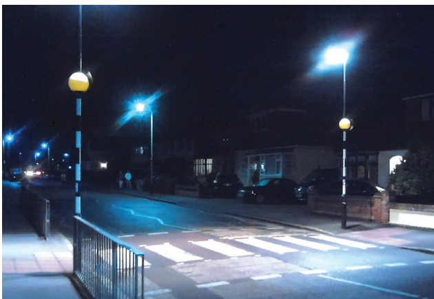
Zebra crossing pedestrian lighting
