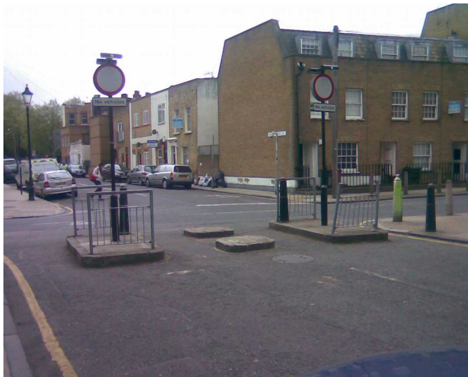
Eric Street, Mile End. Sump breaker.
