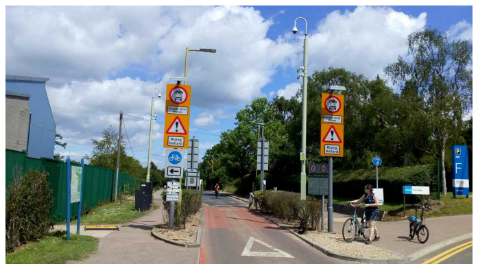
College Lane, Hatfield. Rising bollard-controlled bus gate.
