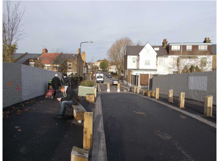
West Avenue, Walthamstow. This railway bridge is essentially a large modal filter which was closed to motor traffic because of structural issues. It's now a place to sit and think as well as walk and cycle through.
