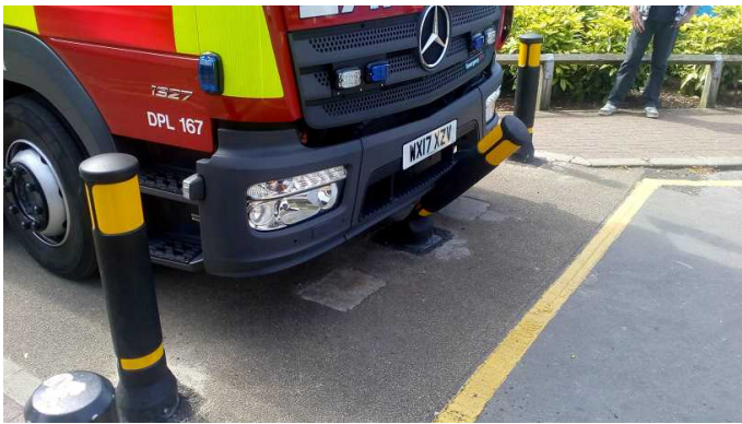
Park End Road, Romford. Collapsible bollard.
