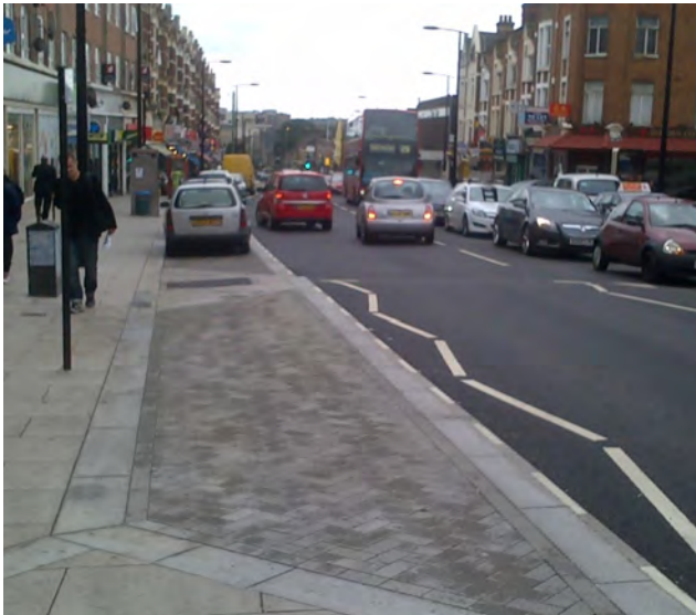
Footway level parking, Sydenham
