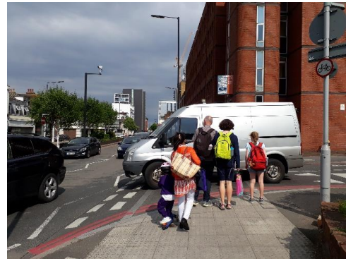
Figure 6: Blended footway, Sutton. Despite the raised table, motorists still assume priority. Photo: Lucy Marstrand
