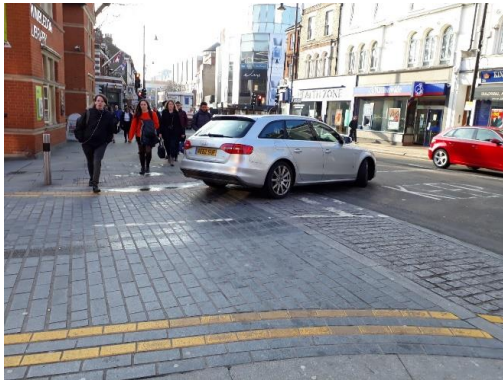
Figure 5: Blended footway: Despite the change in surface material and the raised table the visual priority is still with turning traffic due to kerb line and give-way markings. Wimbledon. Photo: Lucy Marstrand
