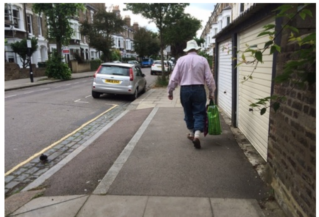
Raised level footway crossovers Roderick Road, London. No adverse camber for people! Cars can handle this.
